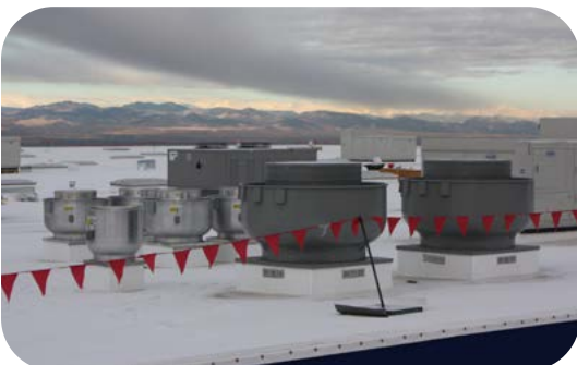
Smoke Exhaust with TCF Model BCRUSH Location: Colorado
