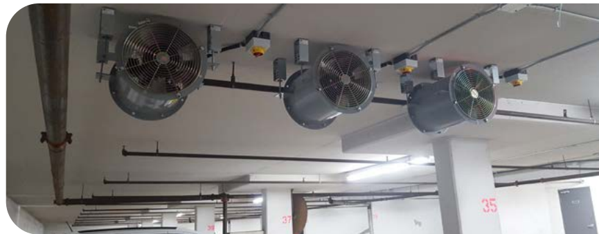
Garage Ventilation with Aerovent Model ATA Location: Canada
