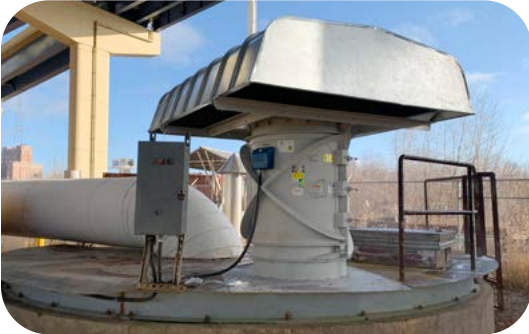
Steam Tunnel Exhaust with Aerovent Model VW Location: Wisconsin
