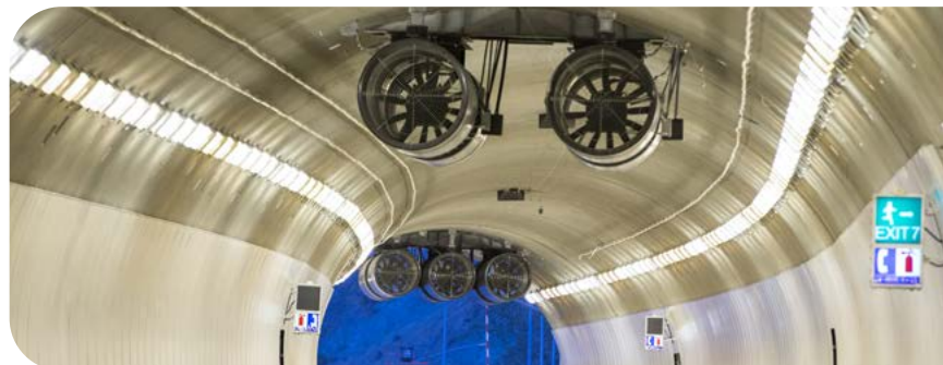
Tunnel Ventilation with Clarage Jet Fans Location: California
